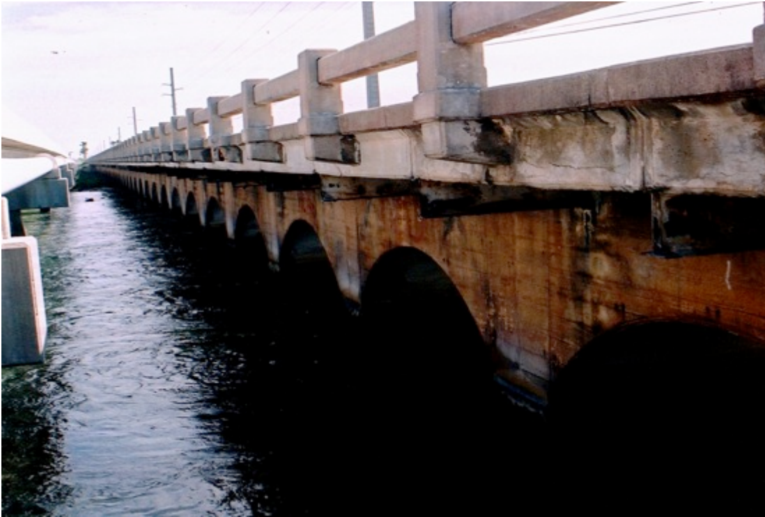
Underside Cast in place repair with GFRP & CFRP bars
