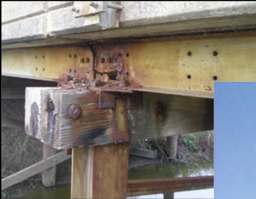
A3015 02-28-06 Span 3, underdeck. Close up of girder deterioration.
