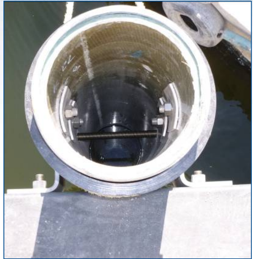
72' PILES, HDPE SLEEVES, FRP INSERT
